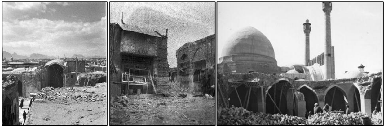
Figure 3. Images of the damaged sections of the Atiq Mosque following the attack by the Iraqi Ba'athist regime (Ashrafi & Abuei, 2024).
