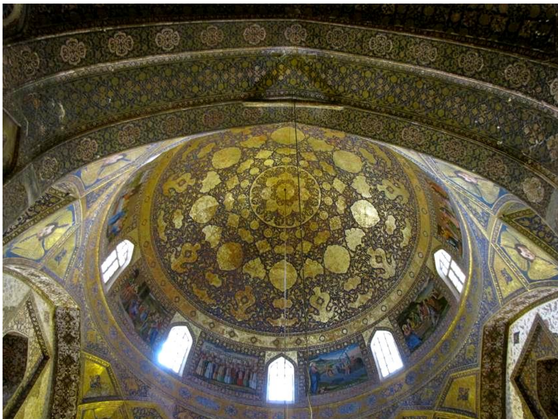
Figure 6. Pastiglia and gilding arrangements in the dome chamber of the Bethlehem Church.
