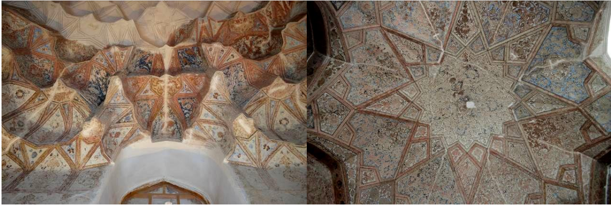
Figure 9. Pastiglia and gilding arrangements in the Mausoleum of Sheikh Jabra'il, Kalkhoran, Ardabil.
