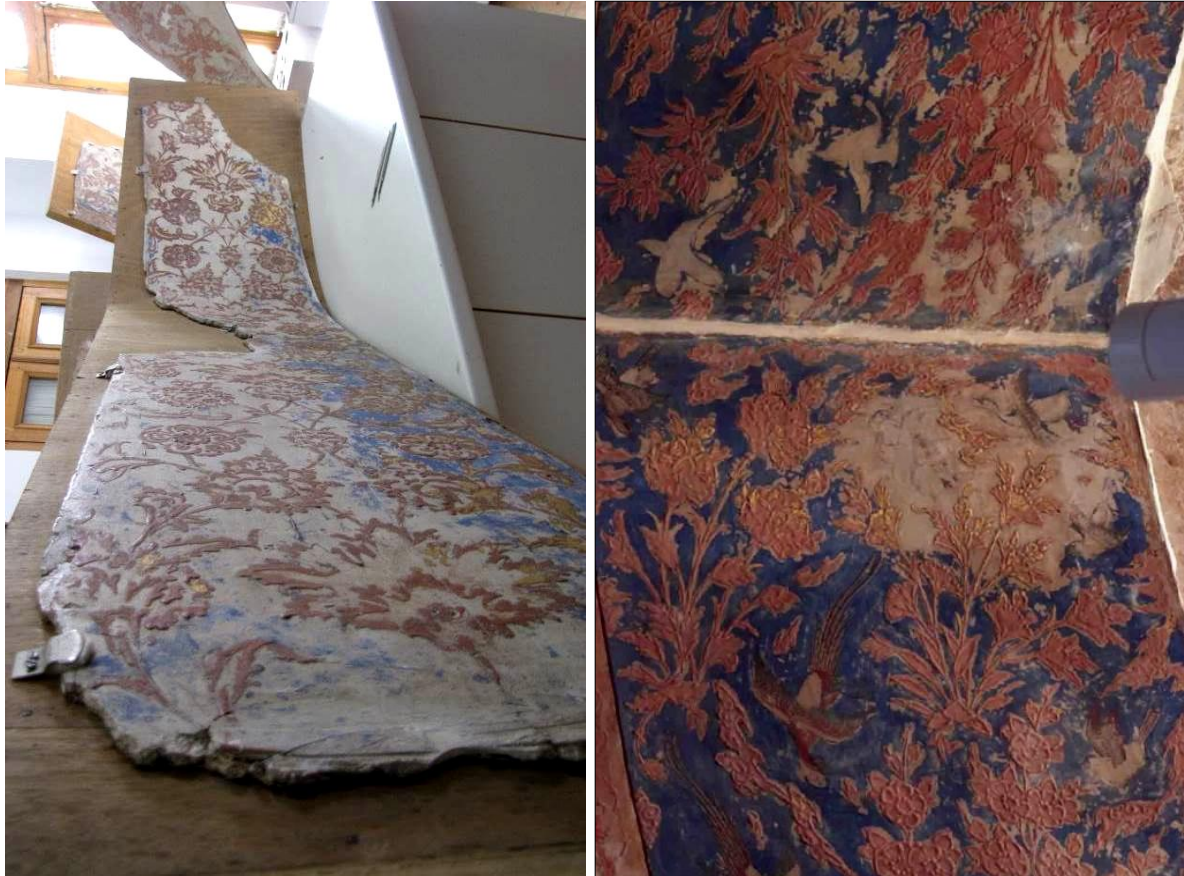
Figure 7. Pastiglia and gilding arrangements (on the building and wooden panel) of the Chehel Sotoun Palace, Qazvin.
