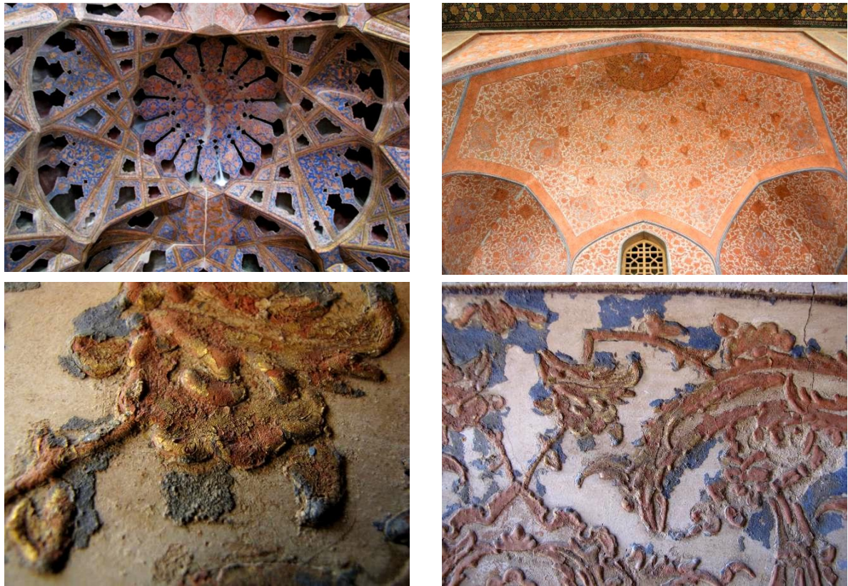
Figure 2. Pastiglia and gilding arrangements on the third and sixth floors of the Ali Qapu Palace, Isfahan.
