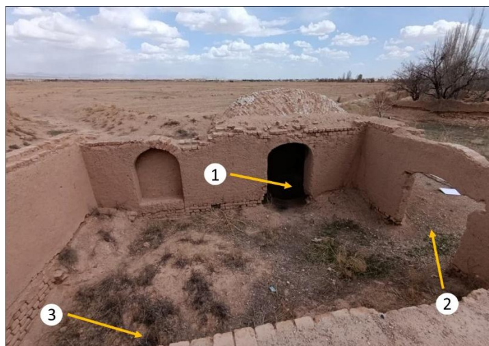
Figure 9. Interior of the western section of the watermill: 1) Door connecting the main room and the storage room; 2) Main entrance; 3) Location of the millstone (photograph taken in 2024).
