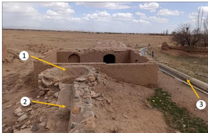
Figure 8. Water inlet path to the watermill: 1) Vertical water shaft (Tanūreh); 2) Channel leading to the hydraulic tower; 3) New water channel (photograph taken in 2024).
