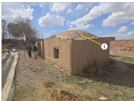
Figure 11. The arch restored in the 2000s (photograph taken in 2024).
