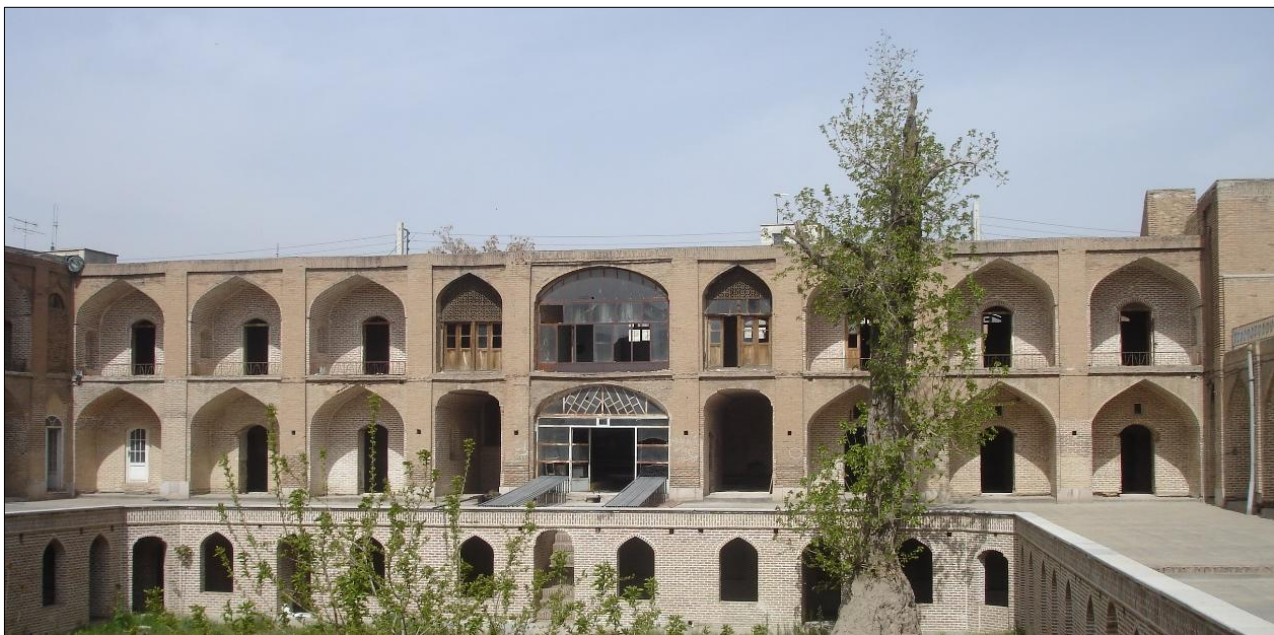
Figure 21. Elevation of Salehiyeh Madrasa—The madras is organized along the east–west axis, located among the student chambers, with arches distinct from the chamber arches (Mazeh-i Kofteh arch) emphasized in the façade.
