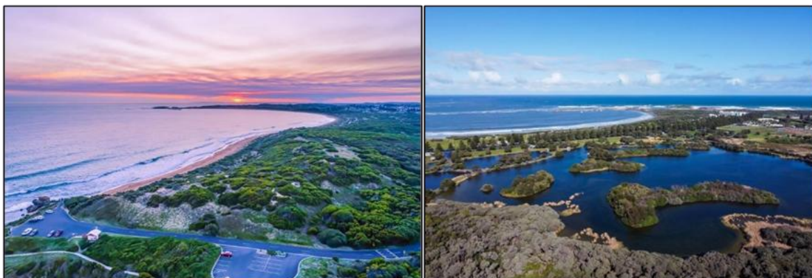
Figure 12. (Left) Revegetation of the Warrnambool foreshore by DEECA, aimed at safeguarding its dune system from erosion. (Right) Lake Pertobe, a scenic tourist attraction in Warrnambool, also functions as a component of integrated water and flood management (Victoria, Department of Transport and Planning, 2025c).
