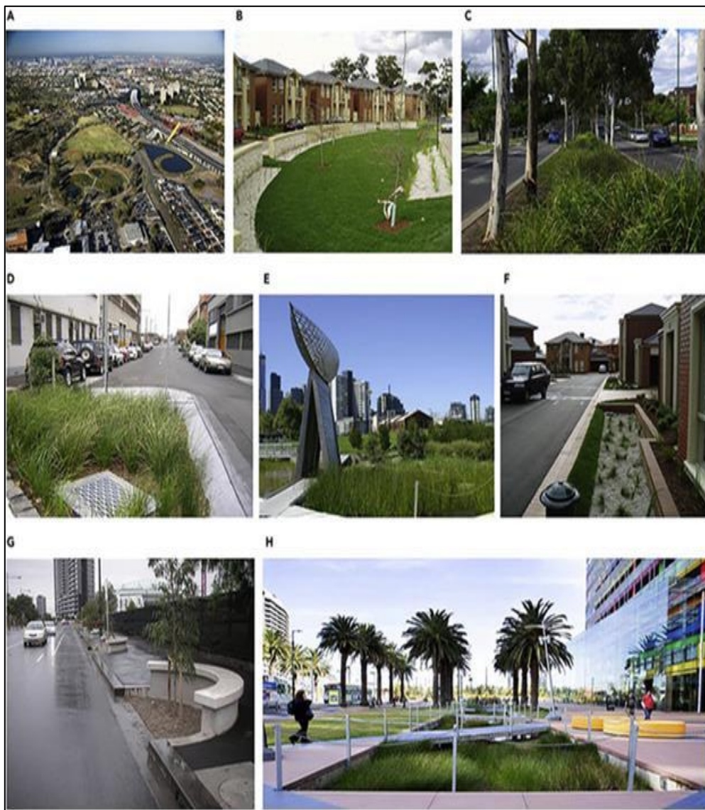
Figure 10. illustrates various water-sensitive urban design strategies for managing surface water retention and flood control through the use of green spaces and permeable surfaces (Wong et al., 2020).
