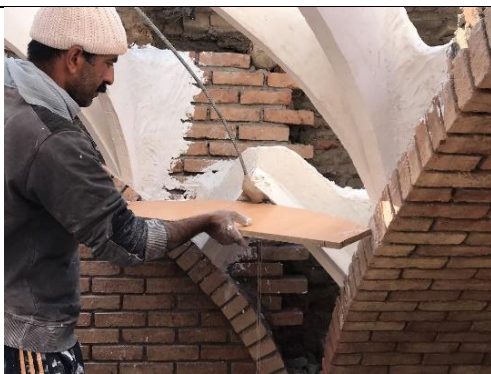
Figure 35: Using bar for the ordering of stretched kite-shaped filler bricks (Timcheh Mirza Jalil Bazaar, Tabriz) (Source: Authors)
