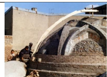
Figure 21: The use of wooden centering for the construction of a domical vault (Tabriz Nobar Bath) (Source: Authors)
