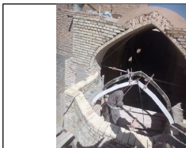
Figure 19: The centerings for construction of the altar primary rib by Mohammad Paknejad (Source: Authors)
