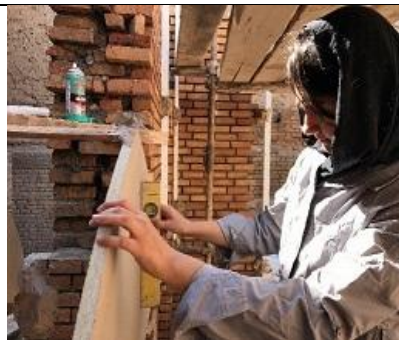
Figure 23: Controlling the plummeting of the mold using a level (Source: Authors)
