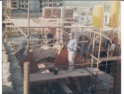
Figure 9: Masonry rib with the mixed brick arrangement (Nabi of Sahand – Tabriz, 2006) (Ref: Authors)
