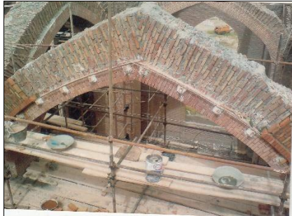
Figure 7: Masonry rib with radial brick vault arrangement (Nabi Mosque of Sahand-Tabriz, 2006) (Ref: Authors)
