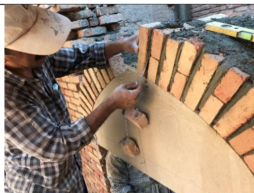
Figure 27: Using nail and cord to control the alignment of the horizontal course of bricks (Source: Authors)
