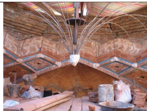
Figure 36: Using bar for domical vault construction (Nabi-e-Sahand Mosque in Tabriz) (Source: Authors, 2006)
