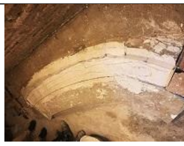
Figure 20: Making gypsum centering (Source: Authors)
