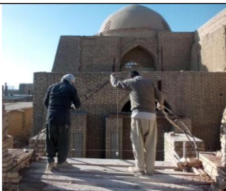
Figure 24: How master-builder plummeting the centering (Source: Authors, 2017)
