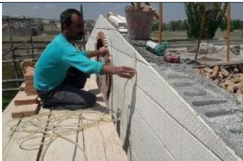
Figure 22: Using a level hose to control horizontal alignment (Source: Authors)
