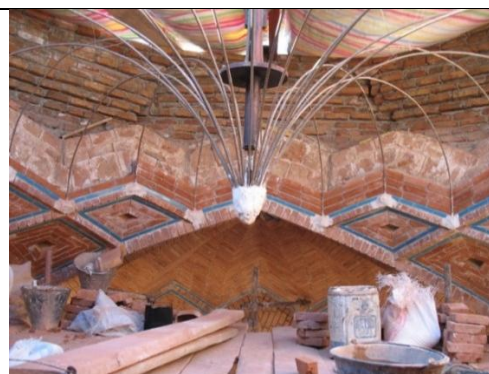
Figure 36: Using bar for domical vault construction (Nabi-e-Sahand Mosque in Tabriz) (Source: Authors, 2006)
