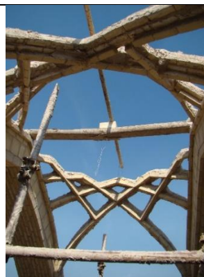
Figure 34: The use of wood and cord to control the horizontal alignment of mold apexes -Bid Abad Bazaar of Isfahan (Source: Isfahan Cultural Heritage Archive)
