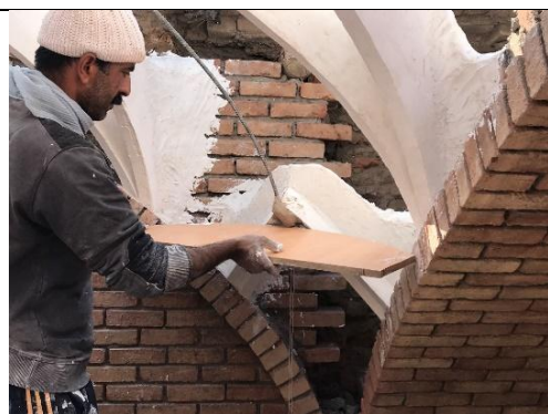
Figure 35: Using bar for the ordering of stretched kite-shaped filler bricks (Timcheh Mirza Jalil Bazaar, Tabriz) (Source: Authors)
