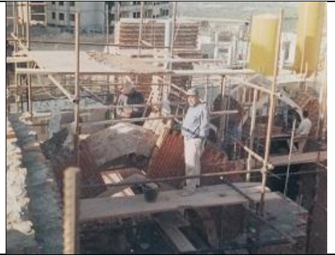
Figure 9: Masonry rib with the mixed brick arrangement (Nabi of Sahand – Tabriz, 2006) (Ref: Authors)
