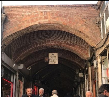
Figure 8: Masonry rib with pitched brick vault arrangement (One of the entrances of Tabriz Bazaar, 2018) (Ref: Authors)
