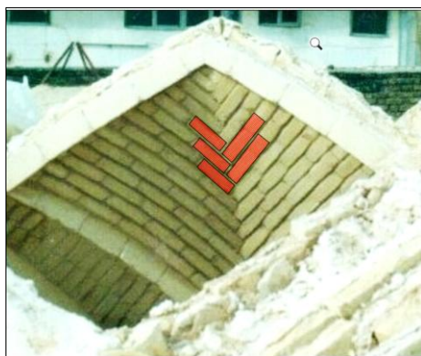
Figure 11: Pa to pa diagonal courses (zigzag form) (Source: Isfahan Cultural Heritage Archive)
